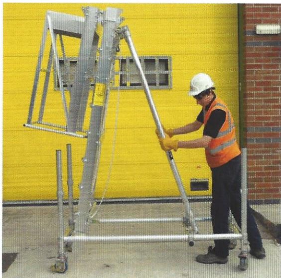
2 From stowed position raise centre section.
