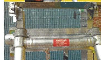
7 Insert dual drop end pins to lock pivoted top section in vertical position. Extend to height if required.
