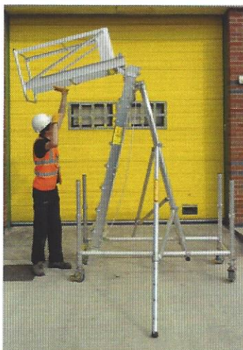
6 Raise cage section keeping arm rigid as ladder is mounted.
